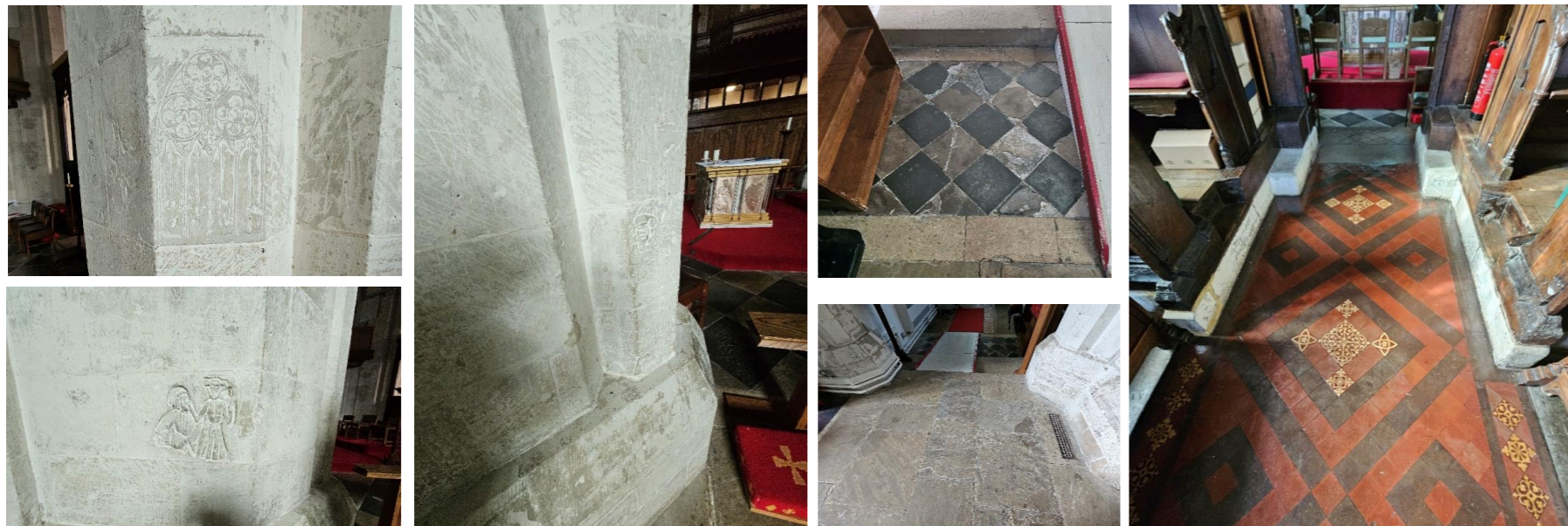
Figure 112 -The abundant graffiti dating back to various stages in the Church's history. The various flooring material ranges from early flagstones (found in the transepts and aisles) to diamond crossing flagstones to Victorian tilework (in the Chancery). NB: the timber flooring next to the pulpit.
