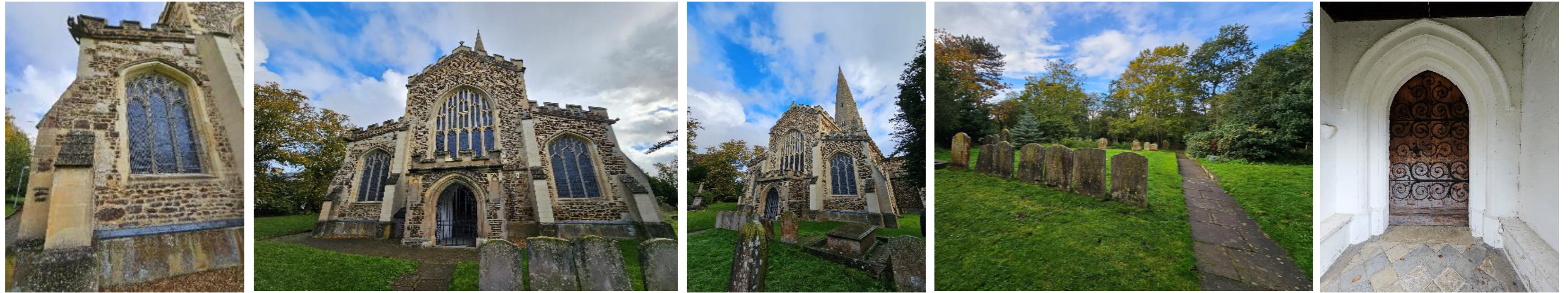
Figure 9-- The western Elevation. Note the equidistant transects and porch additions. All buttresses had been replaced/repared. The graveyard to the west which was extended 4 times (and is full hence the mounding along the north elevation) and the main processional Western doorway which is relatively new but with original ironwork by Thomas de Leighton dated ca C15th.
